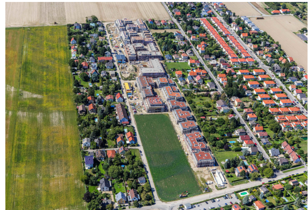
Figure 8 Top view of some municipal districts – left: districts 1, 6 and 7; right: district 22 (Dittelgasse) – for an overview of actual development densities. Source: C. Fürthner
